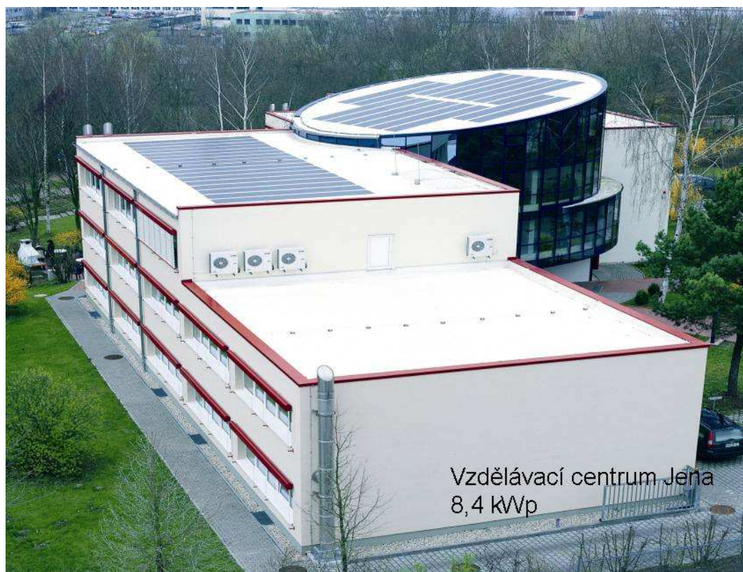
IMAGE 3 Placement of panels on the roof of the Jena educational centre (8.4 kWp)
