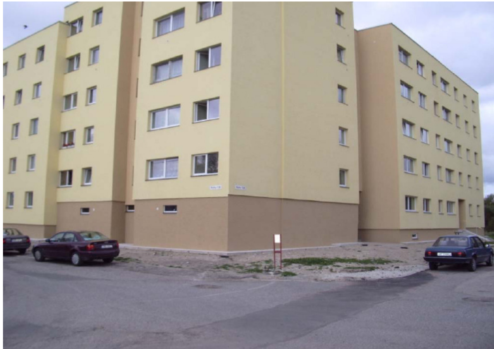
Figure 7: Renovated housing co-operative Estonia
