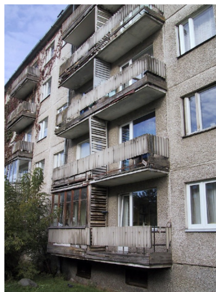
Figure 5: Panel building Estonia
