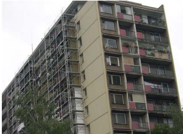
Refurbishment of a building constructed in 1973
