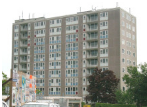
Retrofitting social housing, Belgium (VHM)
